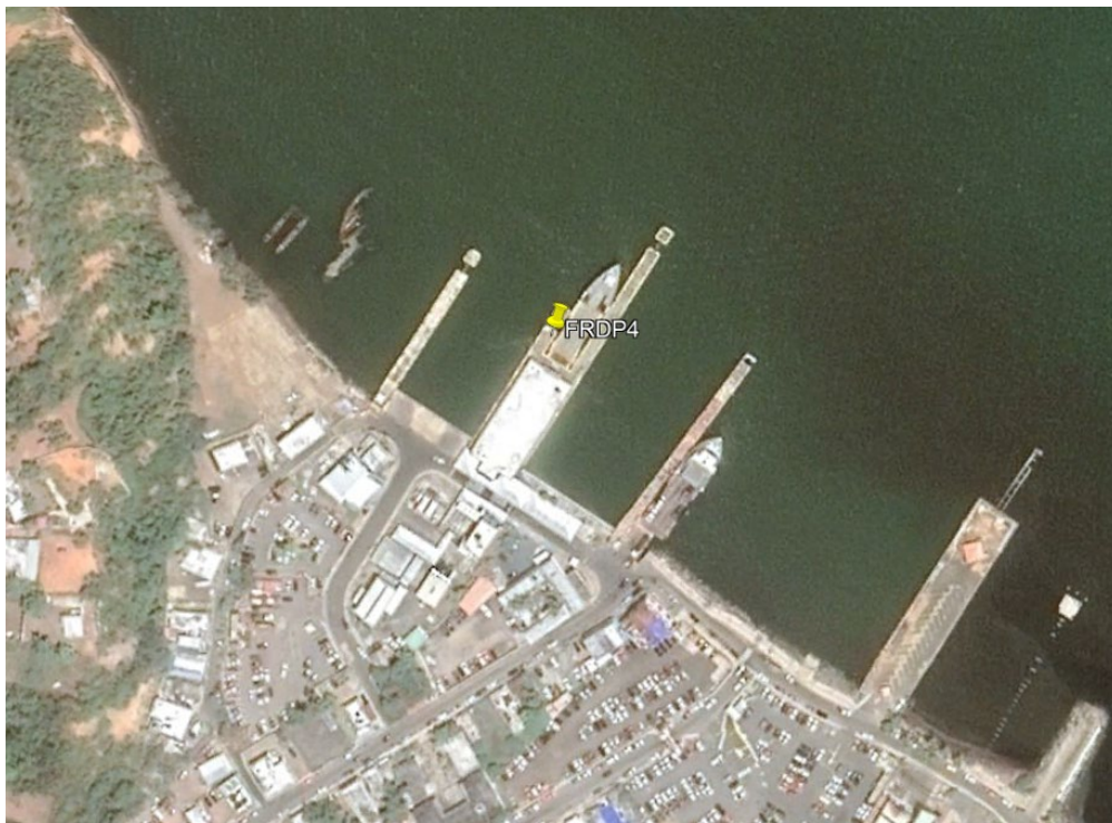
Figure 6-23. Aerial view of NDBC Station FRDP4.
