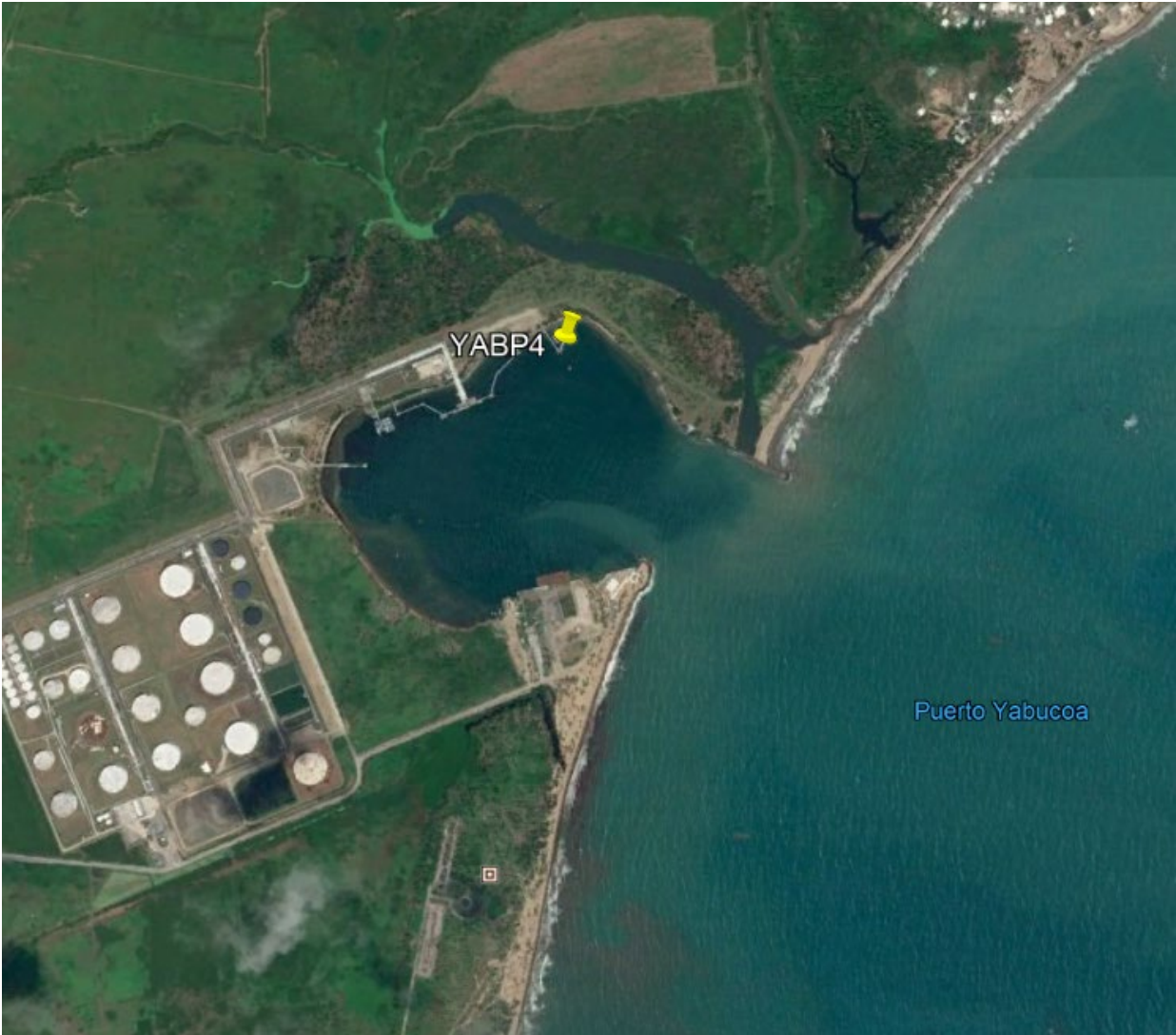
Figure D-12. Aerial image of NDBC station YABP4: Yabucoa Harbor, PR.
