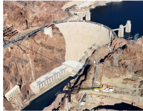
Figure 3-4: An example of a concrete gravity-arch dam is Hoover Dam in the Black Canyon of the Colorado River on the Nevada –Arizona border
