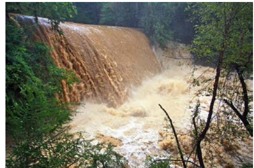
Figure 4-2: Water overtopping the Morgan Falls Dam, GA
